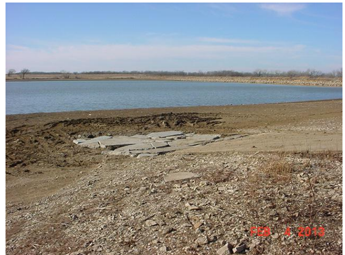
Olpe City Lake boat ramp repair.
